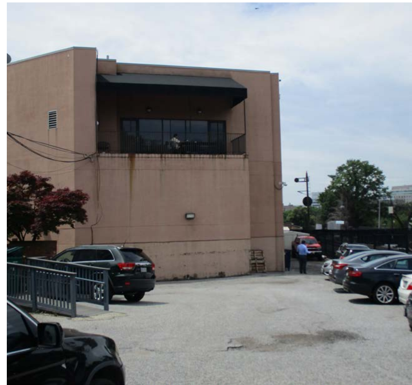
structure in alley to southwest
