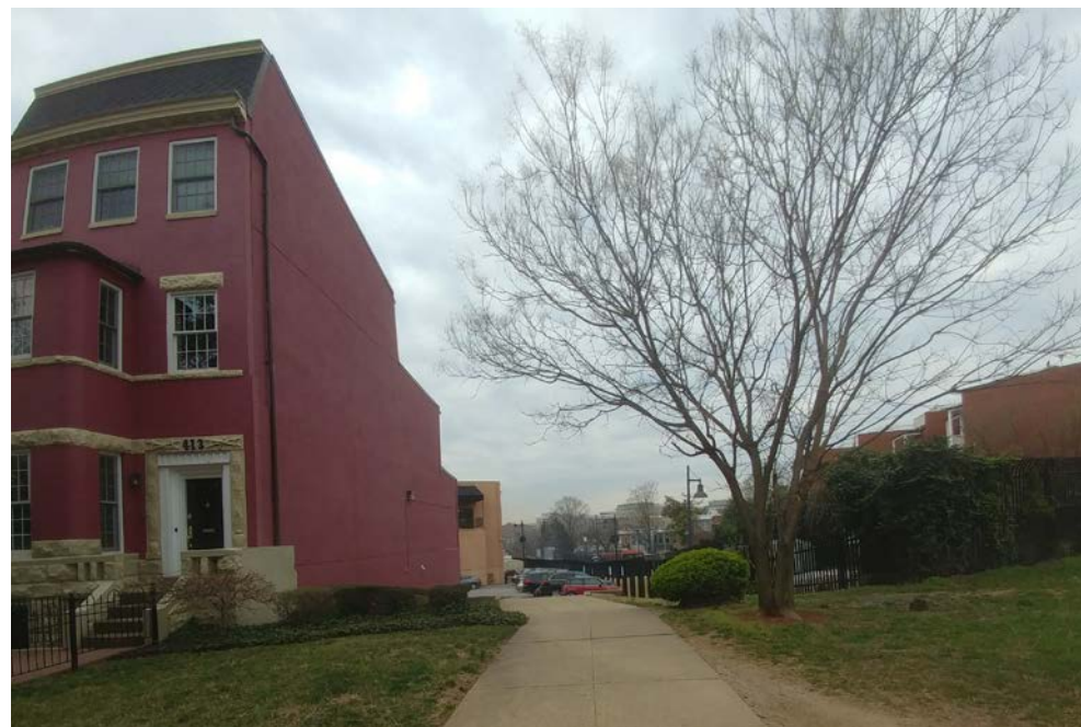
existing condition - street view
