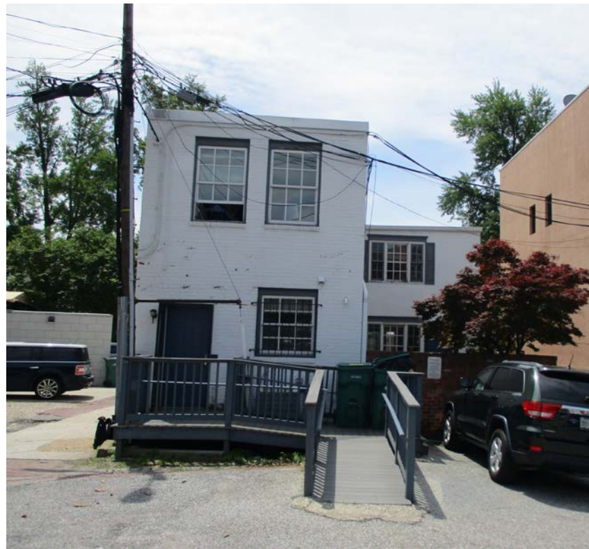
structure in alley to south
